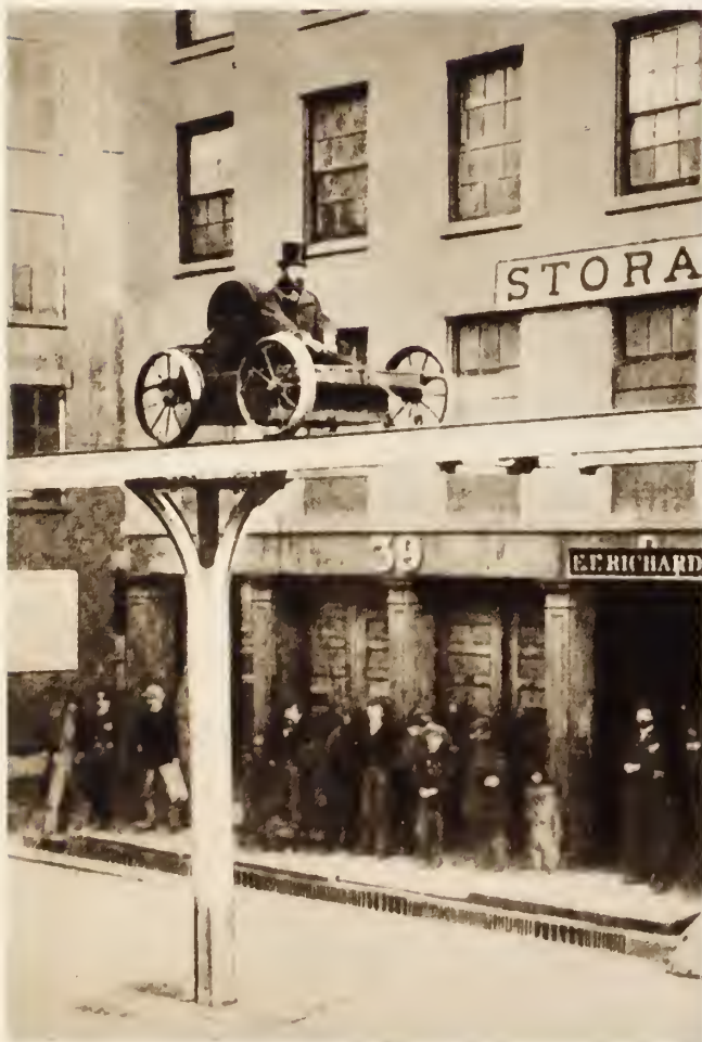
First trip on elevated, to show that train would not jump track.
